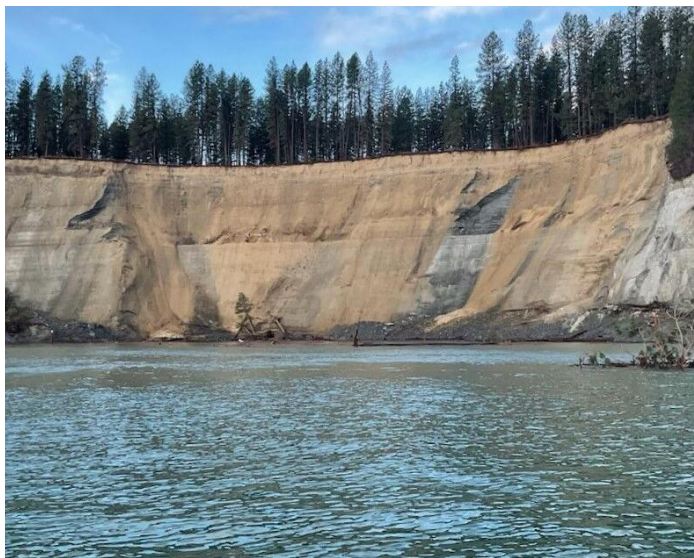
This stunning landslide occurred in November with the area being stable since. Click here to learn more.
