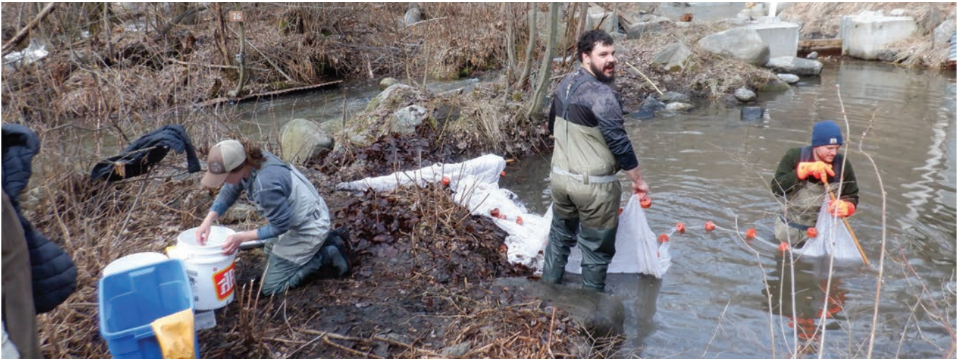
Team at work on Murphy Creek Spawning Channel
