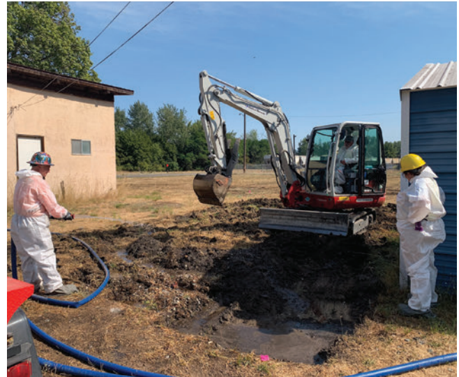
EPA contractor conducting soil removal and implementing dust control measures, with cultural resource monitor present. Northport WA, 2022.
