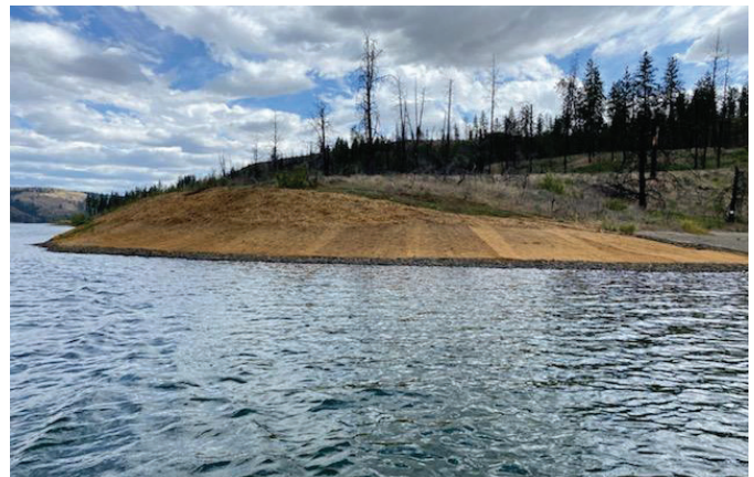
Cayuse Cove phase one construction completed in May 2021
