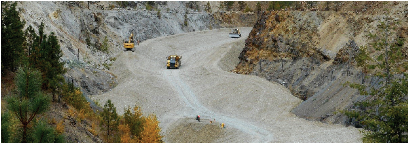
Backfilling the first of two large open pits
