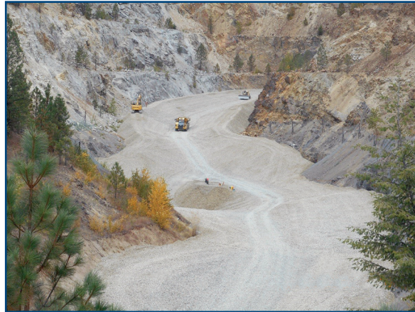
Placing drain rock in Pit 4
