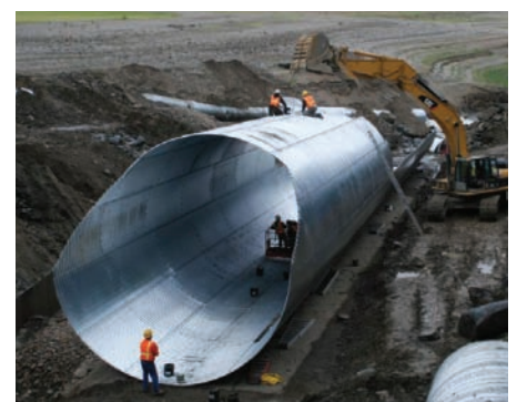
Construction of Barnaby Creek Culvert
