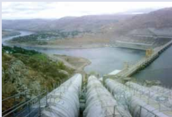
Water is pumped up 280 feet from Lake Roosevelt for delivery to Banks Lake.
