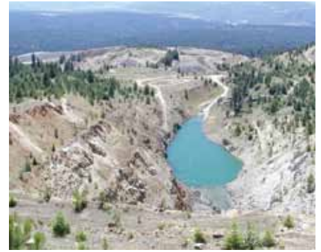
Midnite Mine, Pit 4. This narrow, 500-foot deep pit contains water contaminated by uranium mining.
