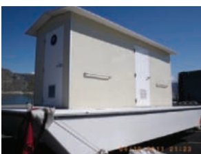
Floating restrooms and pump-out boat
