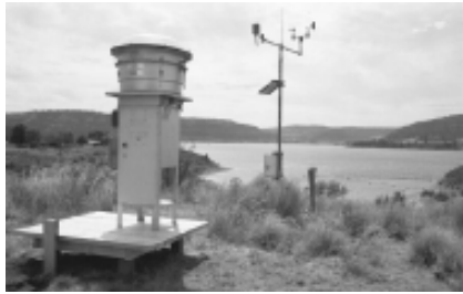
Seven Bays air monitoring station.
