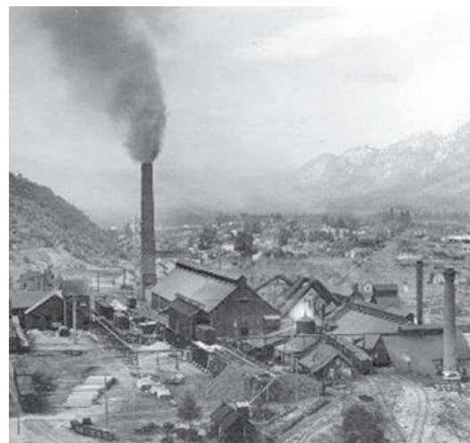
Historical photo of LeRoi Smelter, Northport, Washington.
