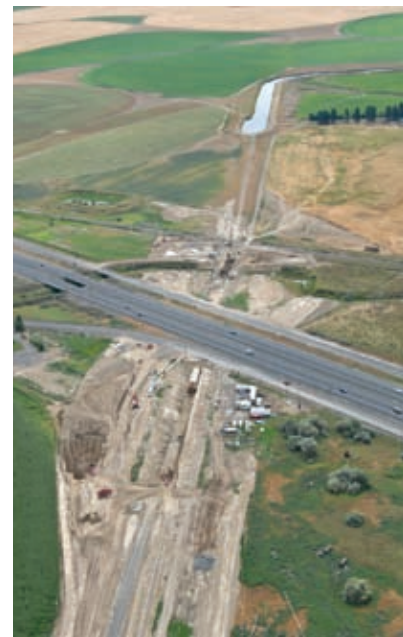
Weber Siphon at I-90
