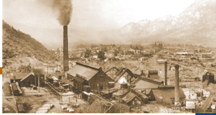
LeRoi Smelter, Northport, WA
