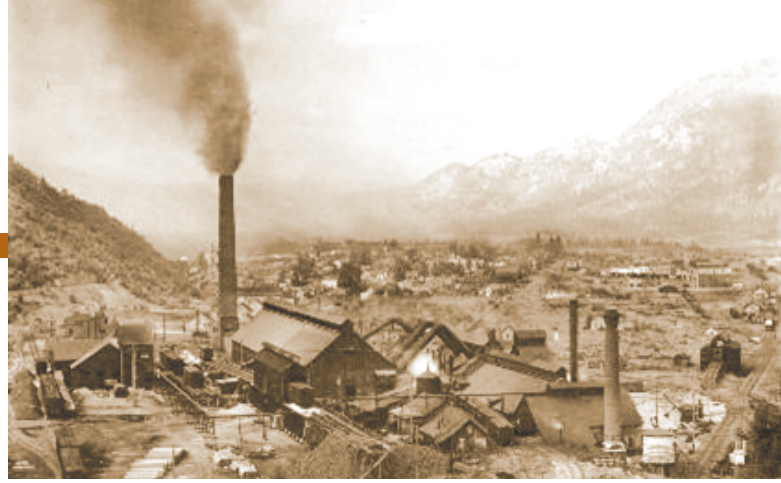
LeRoi Smelter, Northport, WA
